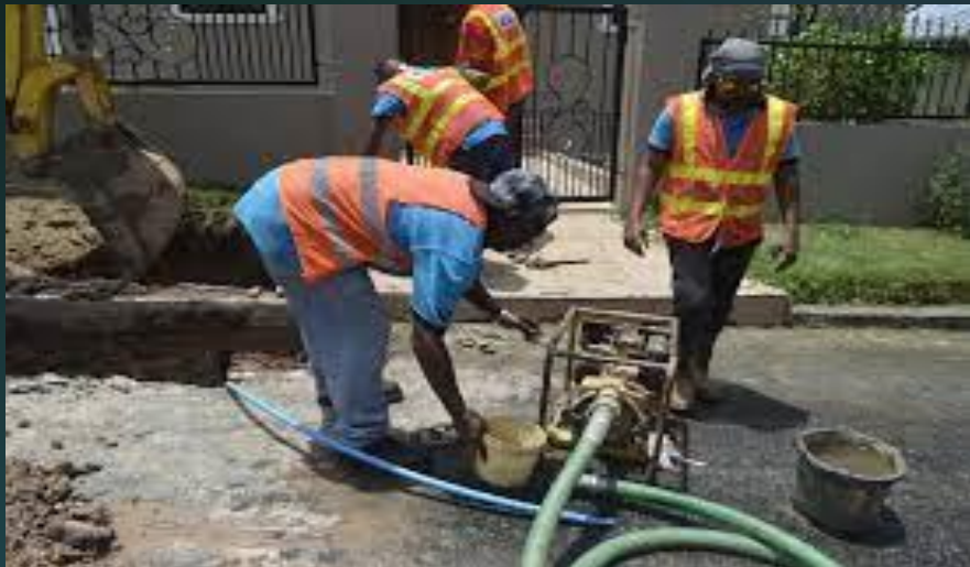
Leak Repair– WASA
